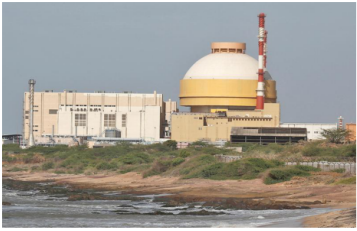
The reported data leak comes amid construction of four VVER reactors at the plant. FILE PHOTO
