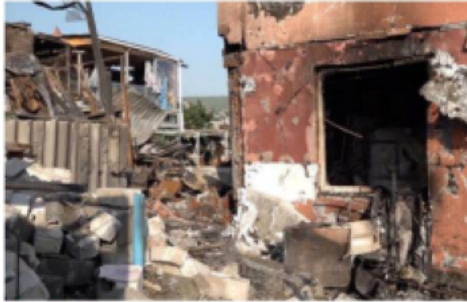
Extensive loss: A damaged private house following a Ukrainian drone strike in Novorossiysk in Russia on Wednesday. REUTERS
