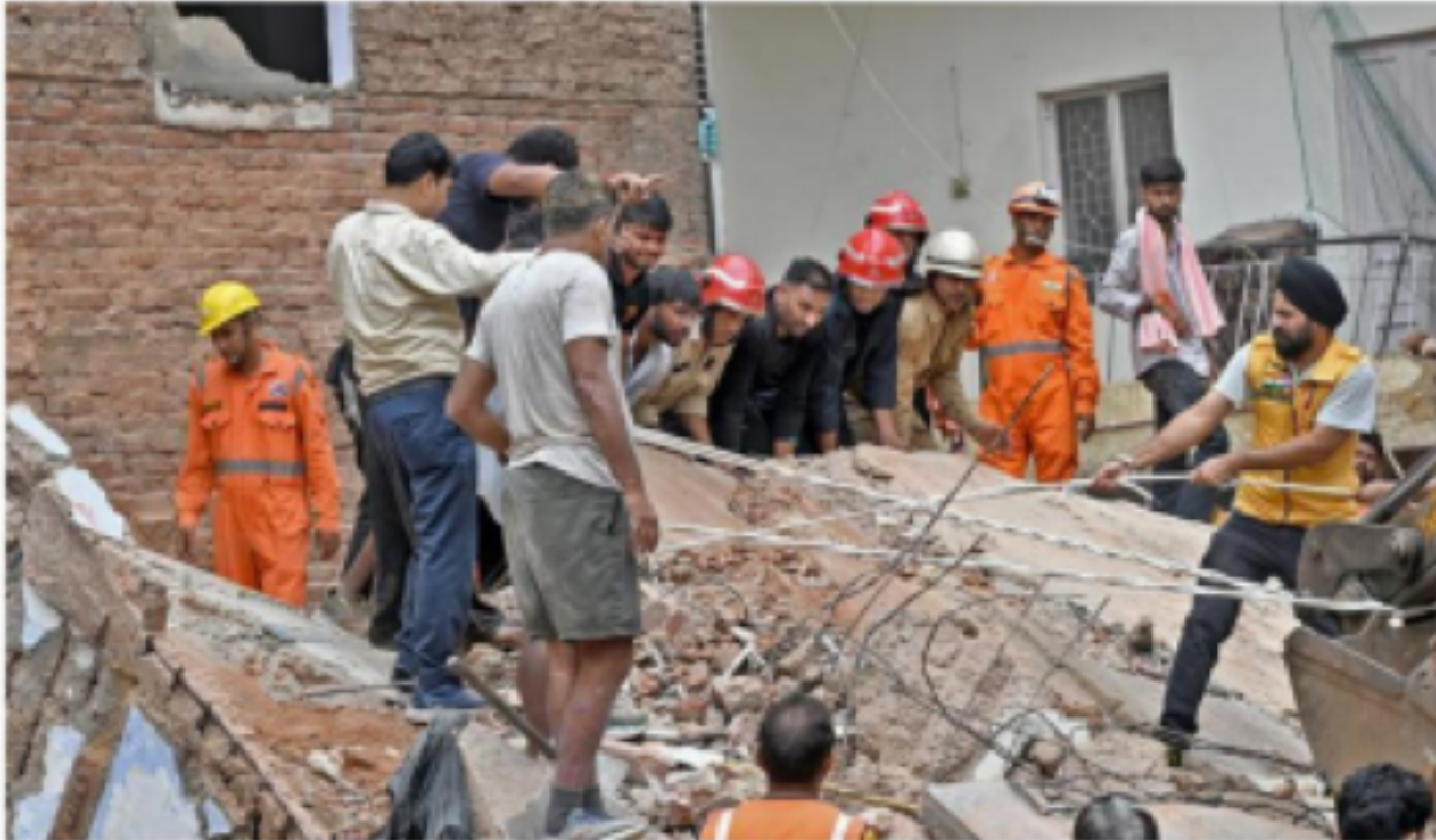
Rescue operations underway after a building collapsed near Satya Niketan in New Delhi on Sunday. SIDDHANT KUMAR
