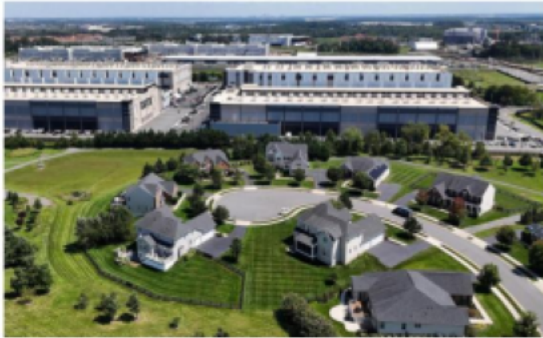
Close encounters: An Amazon Web Services data centre adjacent to single-family homes in Stone Ridge, Virginia, U.S.A.
