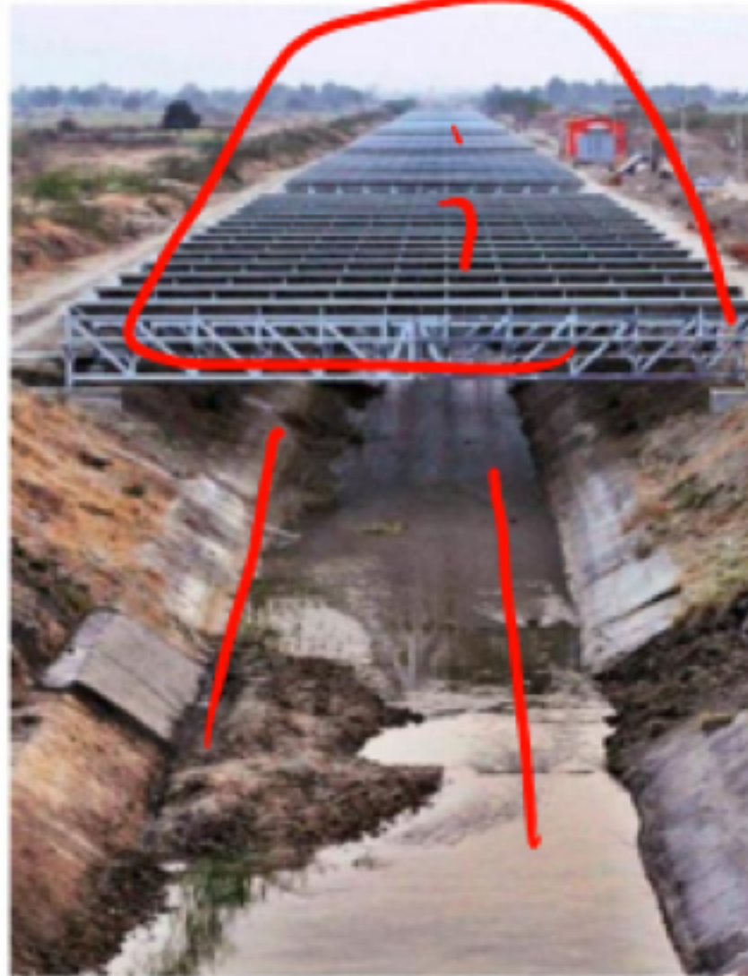
Solar panels seen installed above the Narmada canal in Chandrasan village, Gujarat, in 2012. The State hosted India's first canal-top photovoltaics. AP
